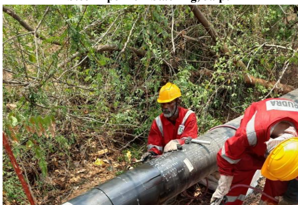
Steel Pipeline – three-layer polyethylene coating, Sangareddy
