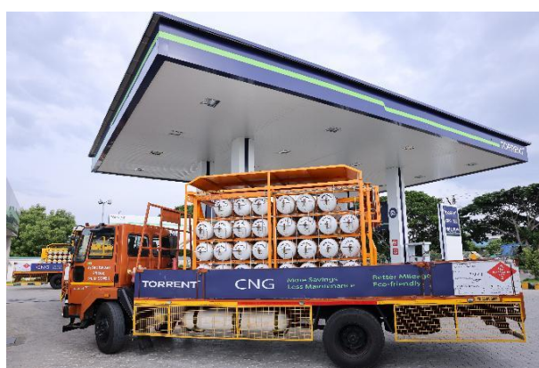
City Gate Station – Cascade Filling
