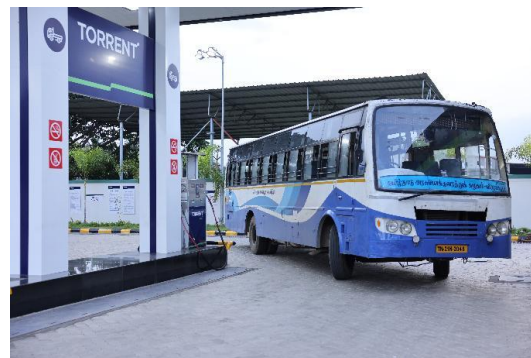
CNG Station, Chennai
