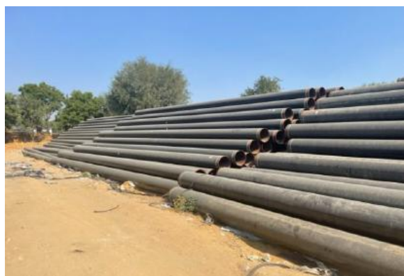
Steel Pipeline – Stacking, Jaipur
