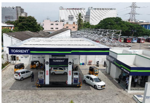
CNG Station, Pune
