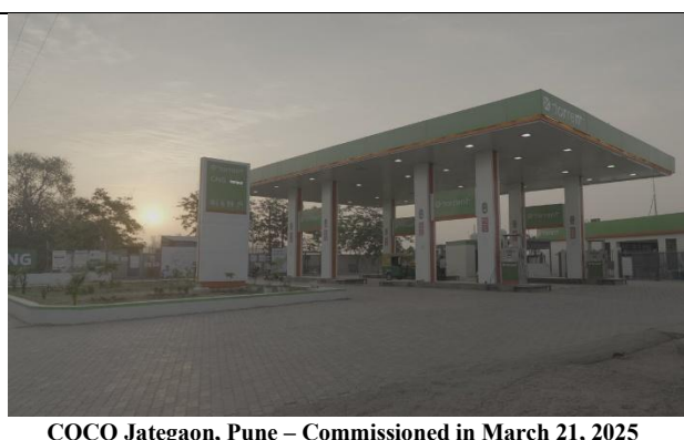
COCO Jategaon, Pune – Commissioned in March 21, 2025
