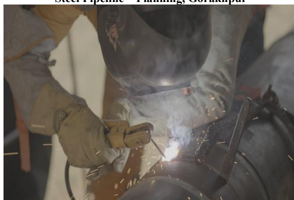
Steel Pipeline – Welding, Gorakhpur
