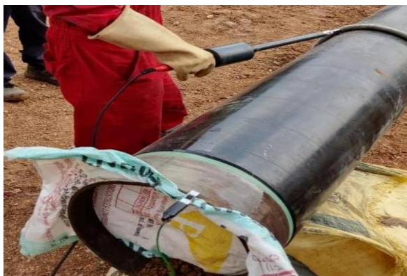
Steel Pipeline – Hydrotesting, Sangareddy
