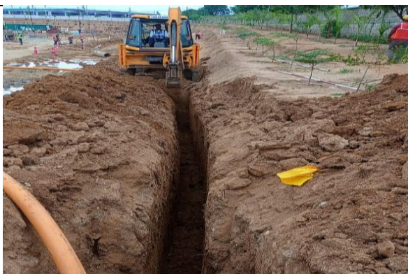
MDPE excavation, Sangareddy
