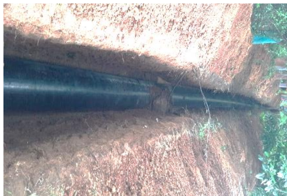
Steel Pipeline – Laying, Sangareddy
